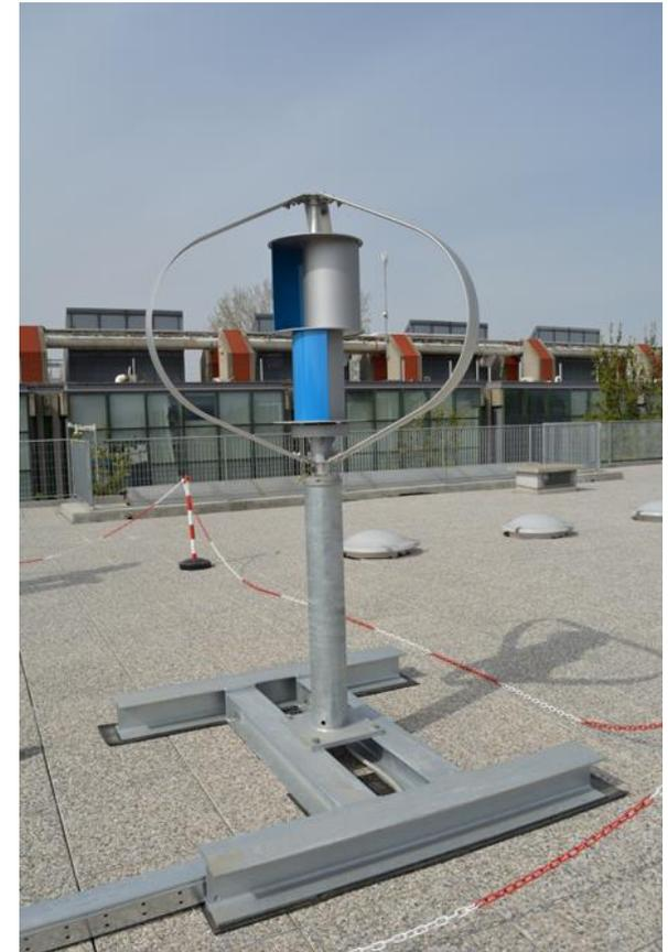
The pole of the vertical axis wind generator must respect the design of the connection flange of the generator itself, it is possible to make self-supporting poles with iron structures to avoid drilling the roof.
